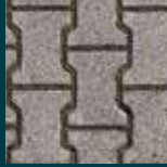
INTERNAL ROADS INTERLOCKING BLOCKS/ TREMIX CONCRETE ROAD
